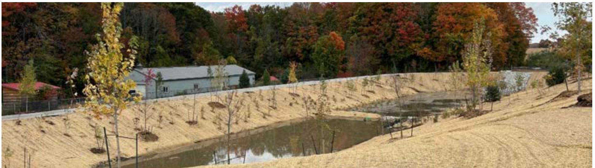
Coral Woods Stormwater Pond
