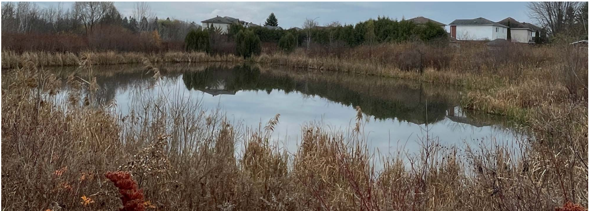
Stormwater Management Pond
