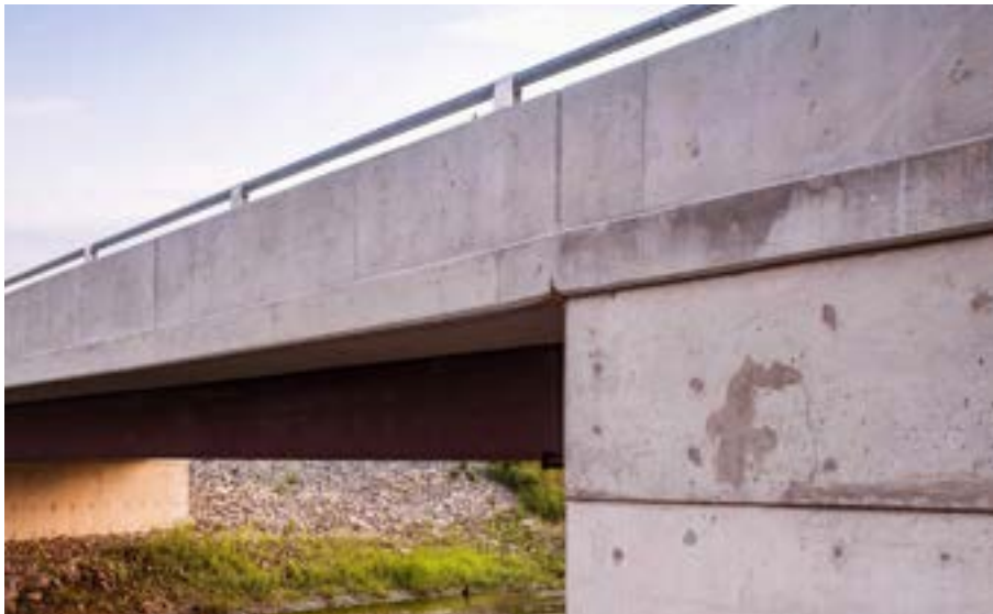
Reive Boulevard Bridge
