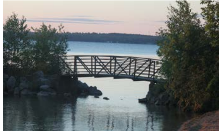
Pedestrian Bridge at Innisfil Beach Park
