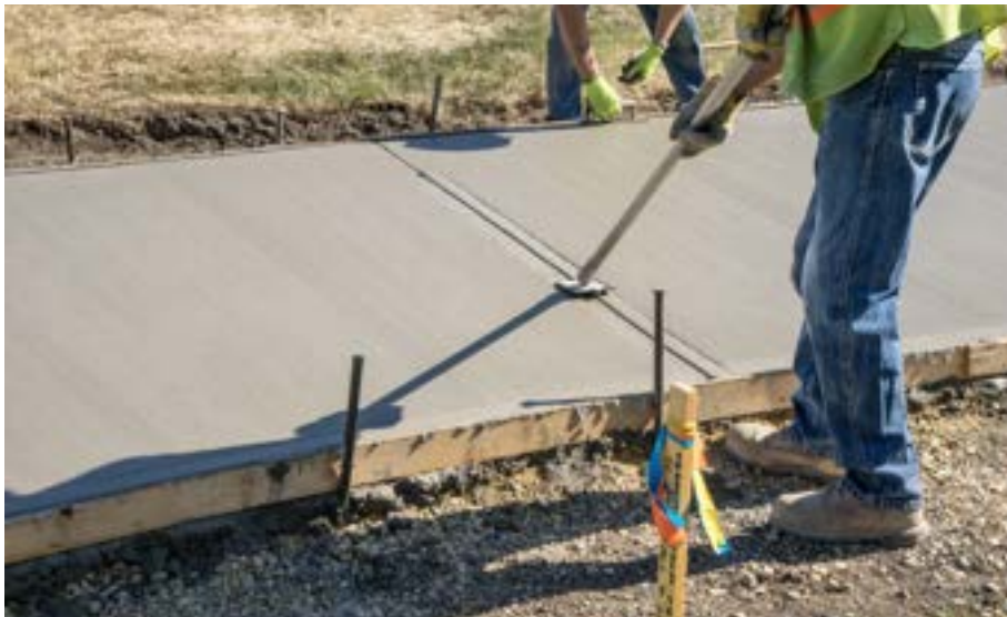
Construction of a concrete sidewalk
