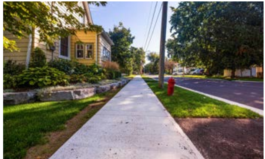
Concrete sidewalk in Cookstown
