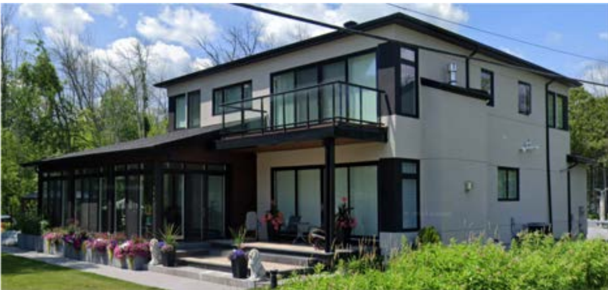
Figure 2 - 974 Barry Avenue at Cumberland Street, Innisfil
