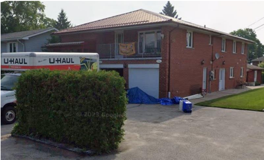
893 Frederick St. is across the street from 900 Frederick St. and it is another large development containing two units with their own attached garages.
