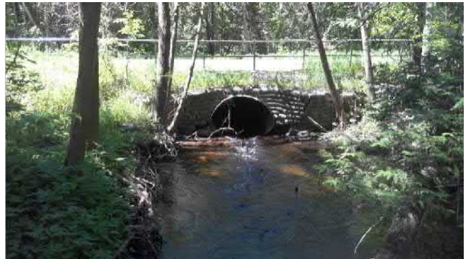
Photo 6. Downstream end of culvert conveying stream under 25 th Sideroad.
