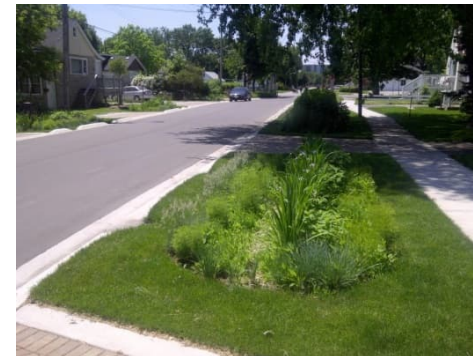
Roadside bioretention facility
