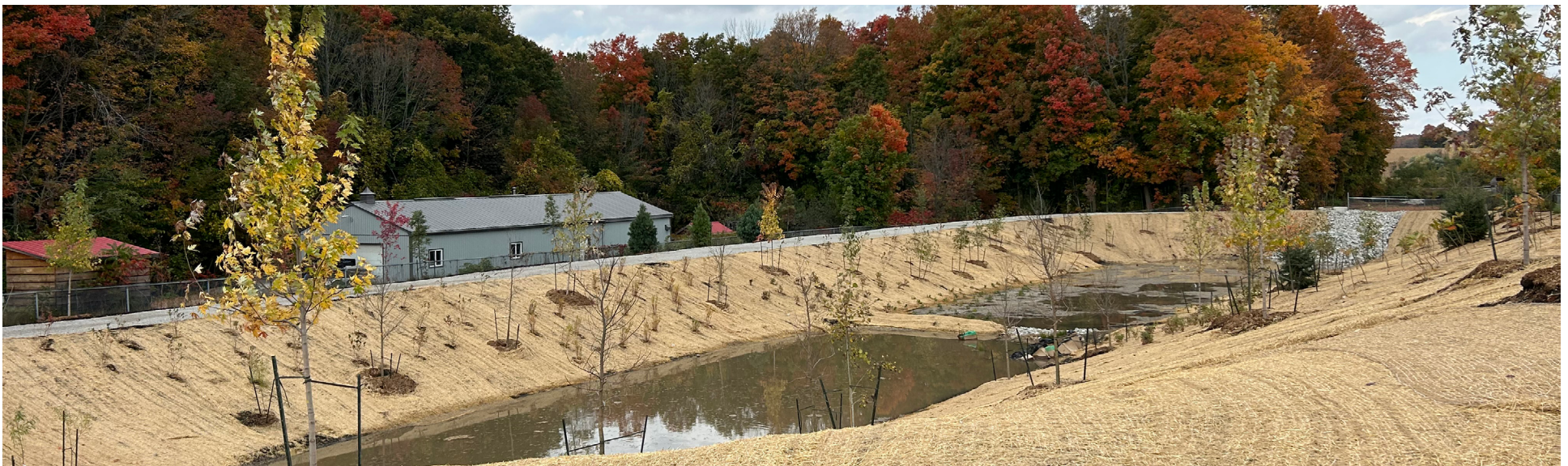
Coral Woods Stormwater Pond
