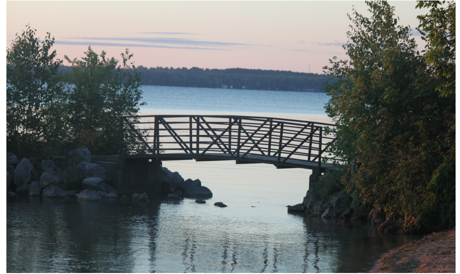
Pedestrian Bridge at Innisfil Beach Park
