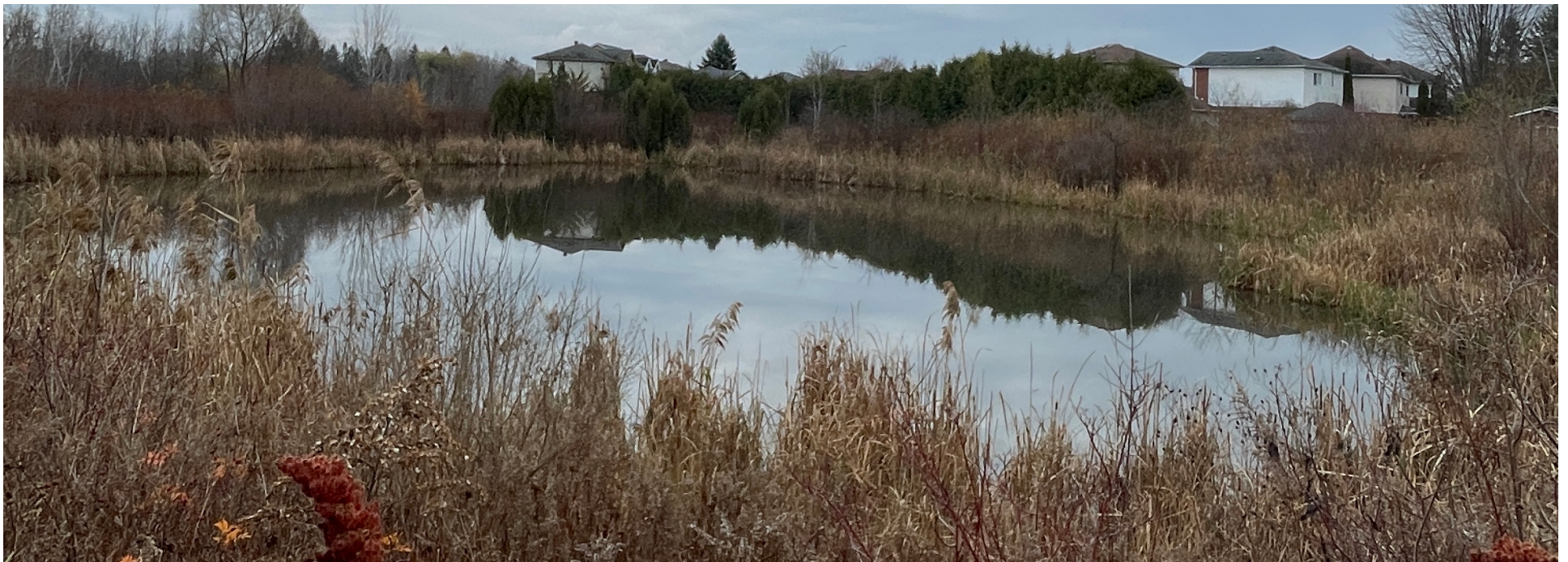
Stormwater Management Pond
