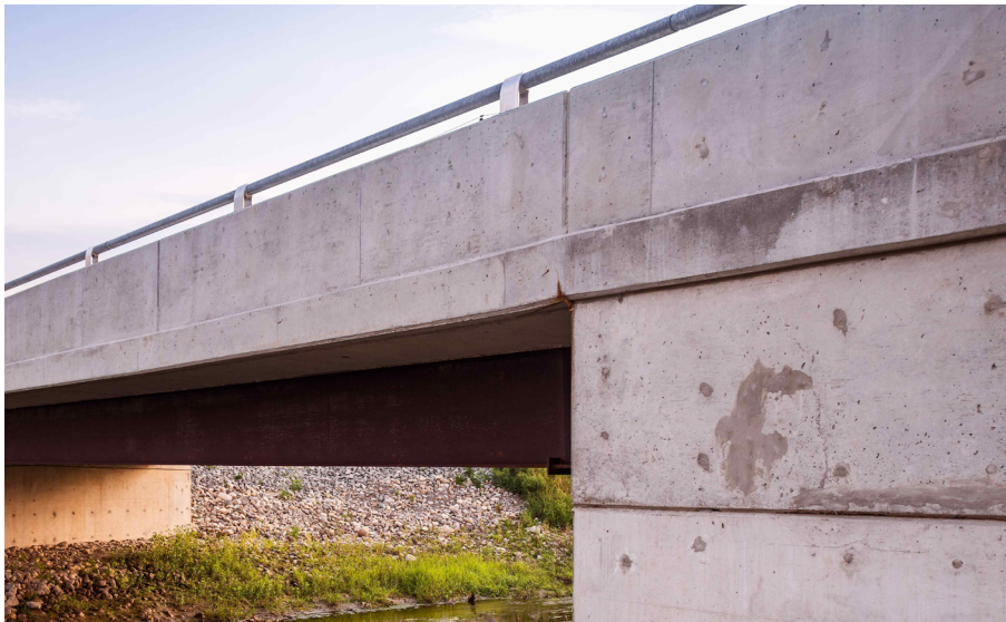
Reive Boulevard Bridge
