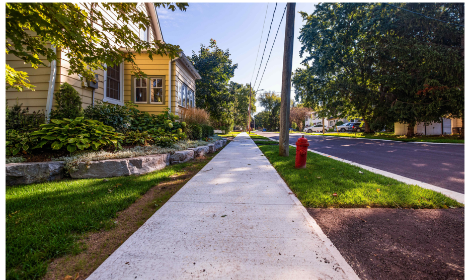
Concrete sidewalk in Cookstown
