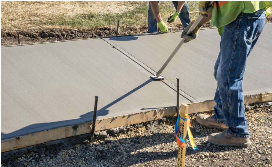
Construction of a concrete sidewalk
