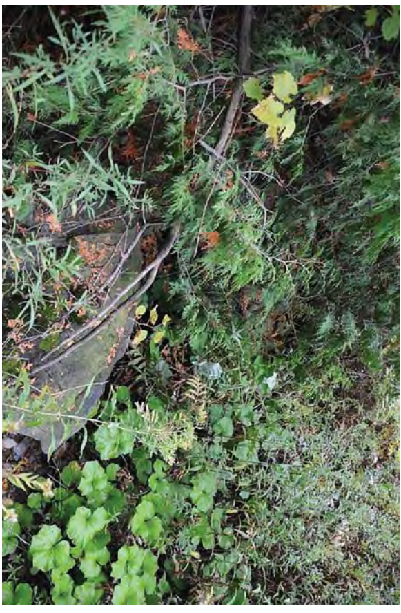
The channel flows down a rocky incline beneath the cedars before connecting with the main channel. It is difficult to determine whether fish passage is available
