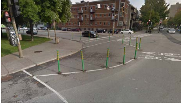
Exhibit 26: Protected Intersection in Montreal, Quebec
