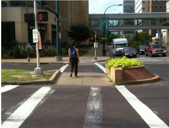
Exhibit 14: Pedestrian Crossing Island
