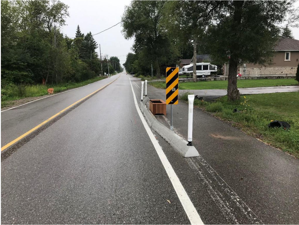
Figure 3: Chicanes at Belle Aire Drive
