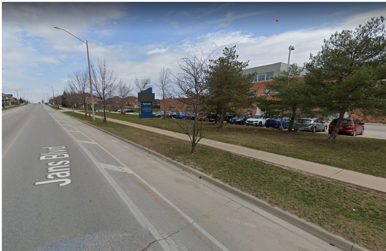
Figure I-1: Cycle lanes along Jans Boulevard (Source: Google Streetview, Image Captured in 2021)
